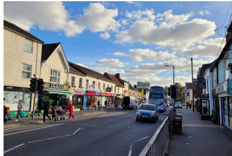
Fig. 15: North Station Road. Views of the southern half of the street (east front).
