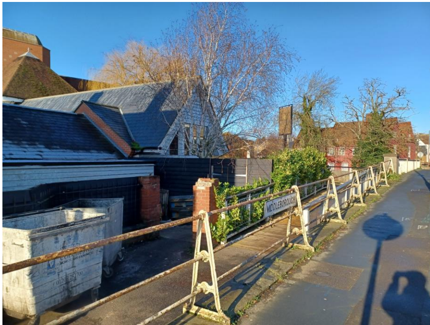
Fig. 48: The historic railings at nos.20-21 Middleborough.
