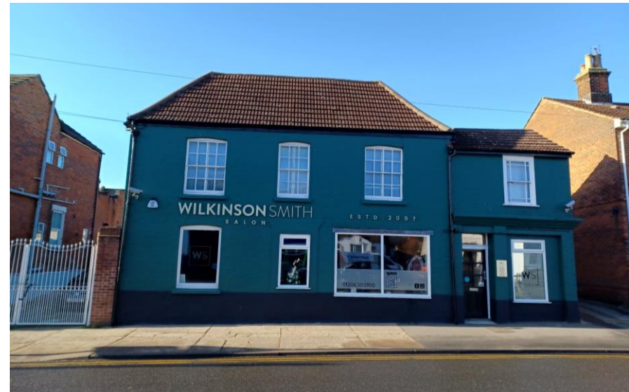
Fig. 70: 66-68 North Station Road.
