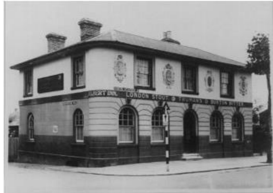
Fig. 50: The Albert Inn, demolished in 1932.
