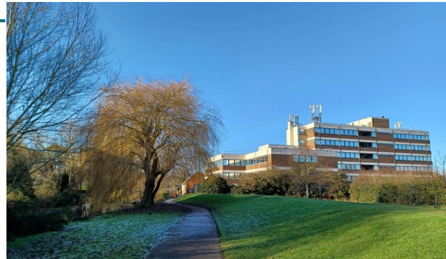
Fig. 33: View from the Riverside walk towards North Bridge to the West.
