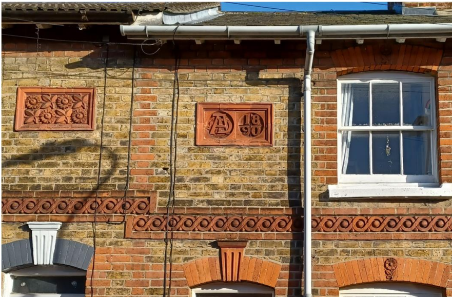
Fig. 77: 1-17 Morten road. Decorative details , including tile with the year of construction (1890) and initials for builder A. Diss.
