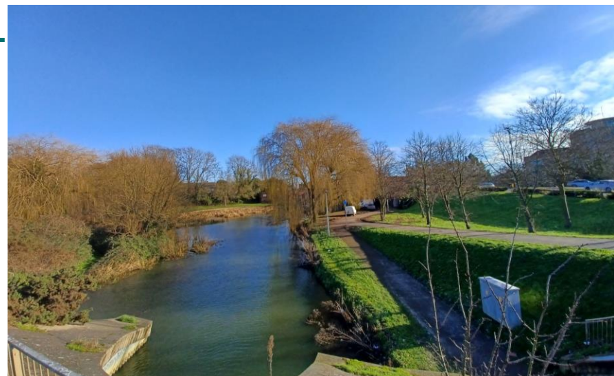
Fig. 25: View of the former Open Air Swimming Pool form the north-west.
