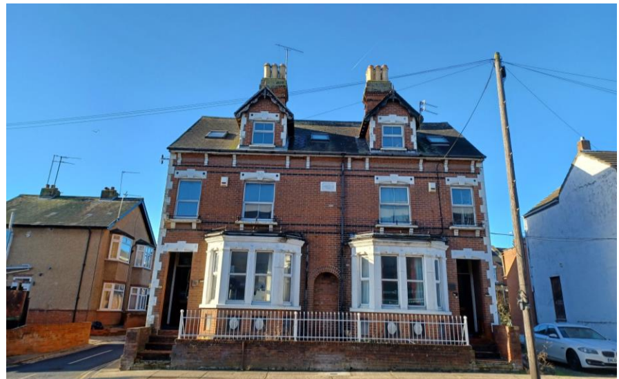
Fig. 71: 60 -62 North Station Road.
