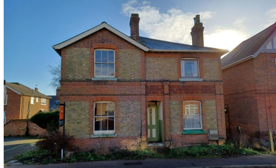
Fig. 78: 25 Morten Road. North elevation (to be replaced with west elevation)
