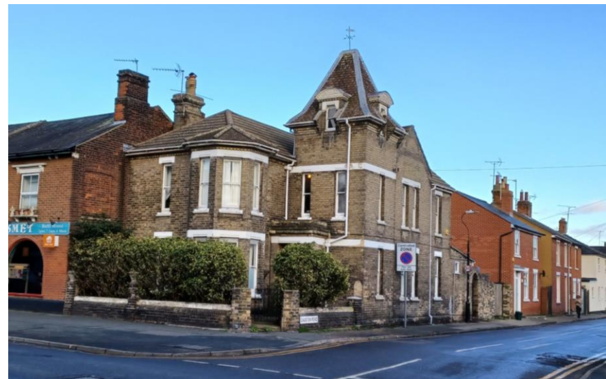
Fig. 60: 29 North Station Road. View from the south-west.
