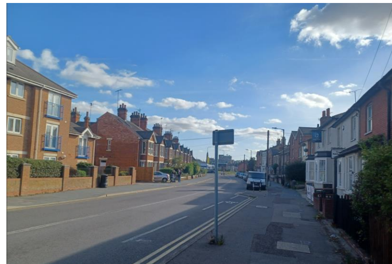
Fig. 14: North Station Road. Views of the northern half of the street (east front).
